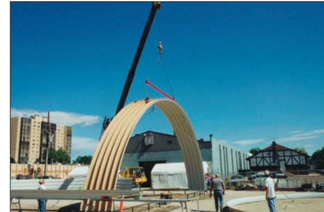
Five curved arches are seamed together on the ground, and set in place on the foundation steel.
