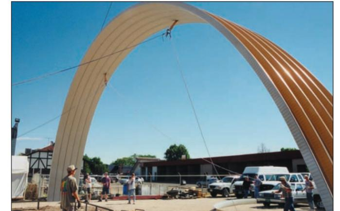
First group of arches are tied off to hanger brackets, plumbed and squared, and welded in place.
