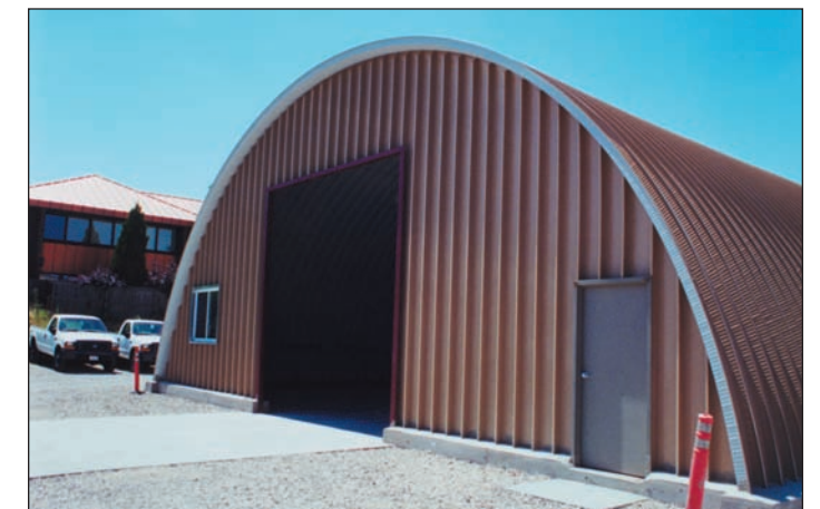
After all panels are welded or fastened to the foundation steel, the end cap is set, and concrete is poured.
